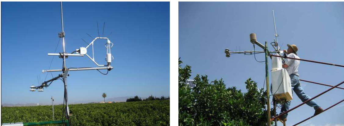
Figure 15. View of the eddy covariance equipment (sonic anemometer, CO 2 and H 2 O analyser) to measure the flow of CO 2 and evapo-transpiration installed by the Universidad de Cartagena.
